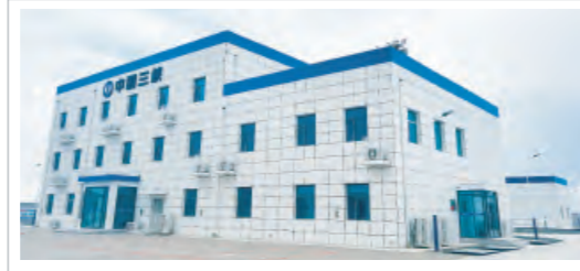
Ulanqab 180MWh Green Power Station Demonstration Project
