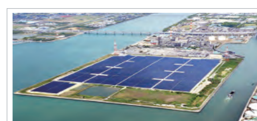
Japan UBE factory in Osaka 6MWh Project
